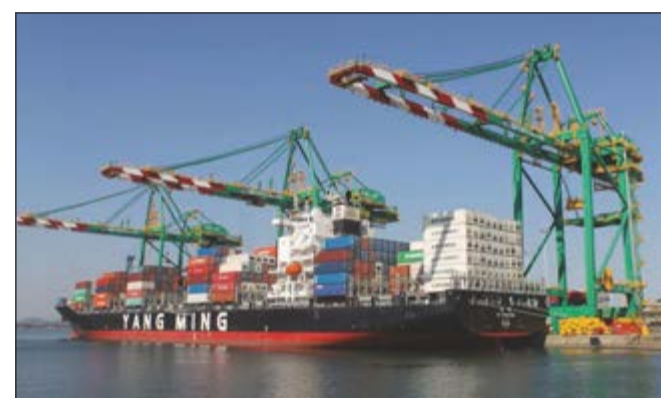
After taking over Tecondi in 2012, EcoRodovias added three STS cranes
