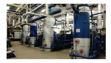
The ammonia heat pump solution has cut process utility costs at the Halifax site by over \$394,000 per year. In addition, the reduction of gas combustion has reduced CO2 emissions by over 1.1 million pounds per year. The Nestlé system recently won the Industrial and Commercial Project of the Year title at the 2010 RAC awards.
